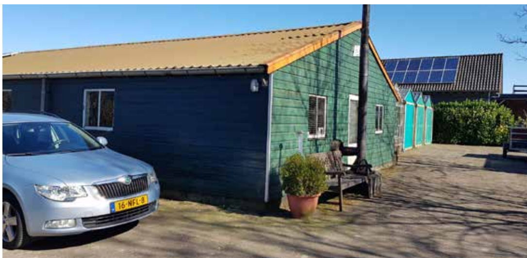
De te slopen loods.
