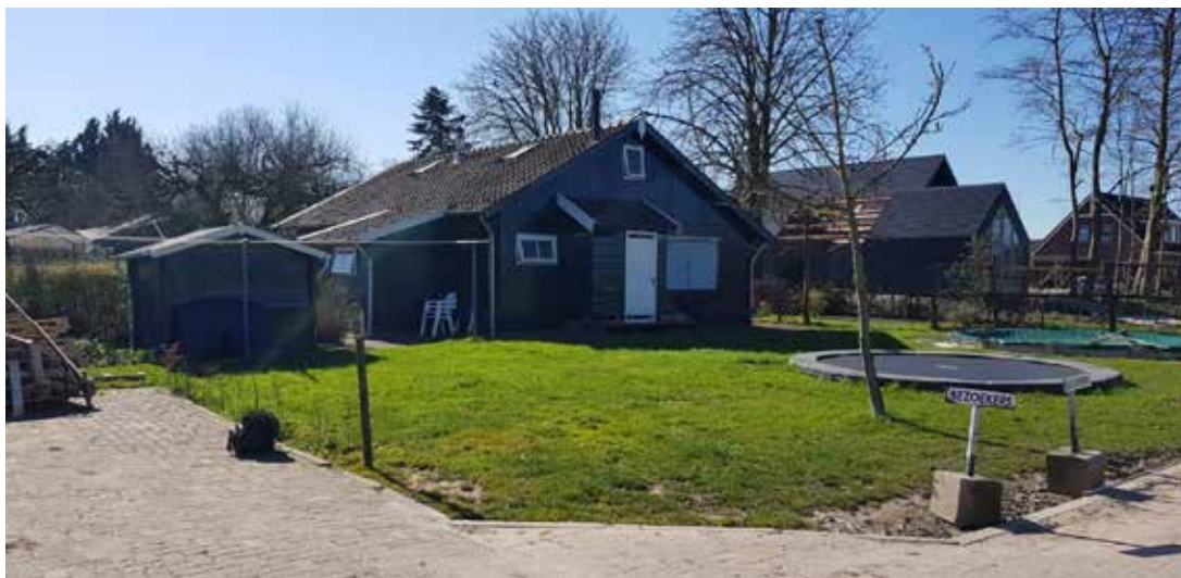
De te slopen woning.
