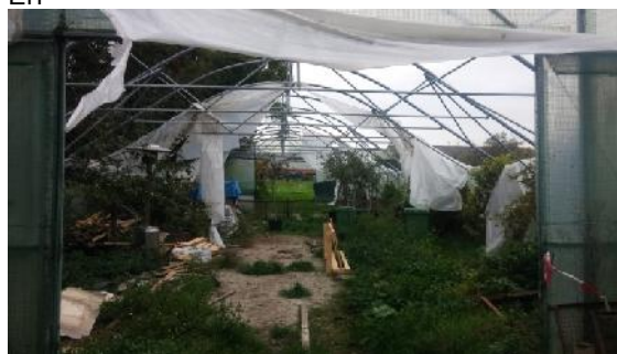
Te slopen tunnelkas
