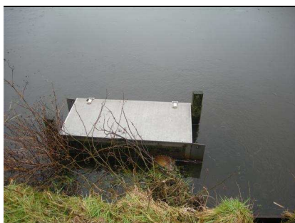
Figure 2.25 Filter box for capturing granules discharged through storm water
