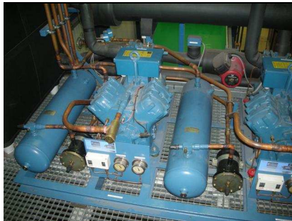
Figure 2.13 Cooling water unit of the injection moulding machines
