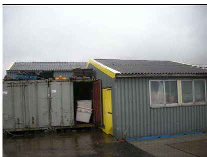
Figure 2.21 Suspected asbestos roofing on the barn and the moulds storage room beyond
