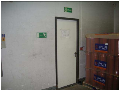
Figure 2.10 Substandard fire door - 2 (no illuminated exit sign - best practice issue)
