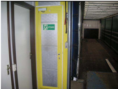
Figure 2.9 Substandard fire door – 1 (no illuminated exit sign - best practice issue)
