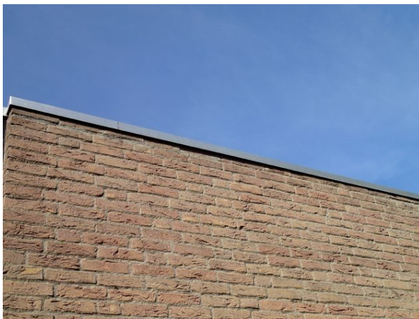
c) kierende aluminium dakrand.
