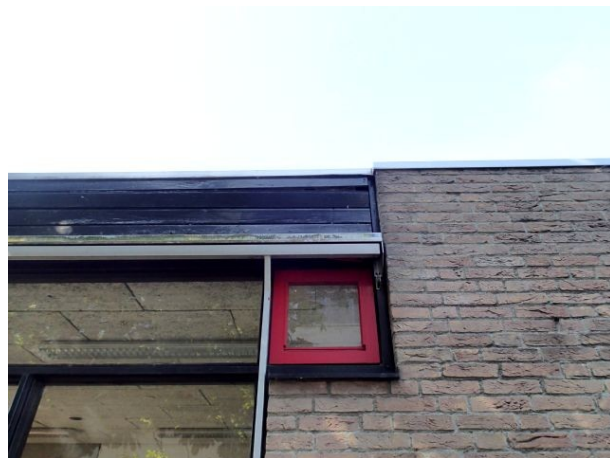
d) loszittende plank van houten dakrand.
