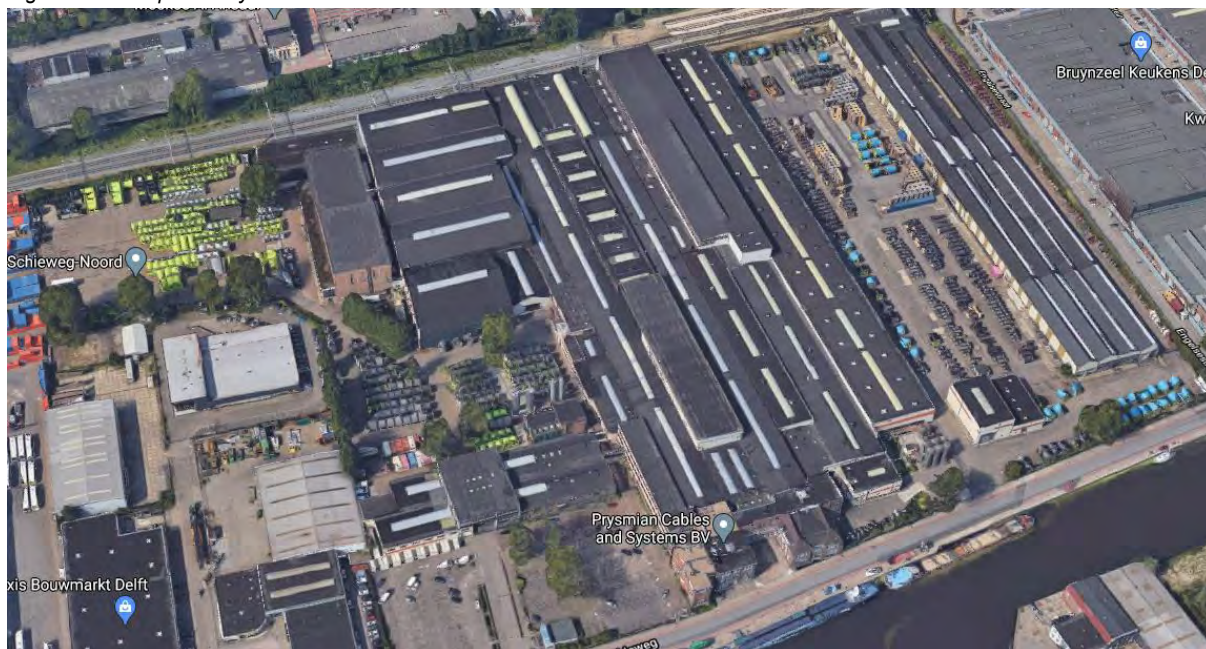
Figure 7: Aerial photo Prysmian from the east
