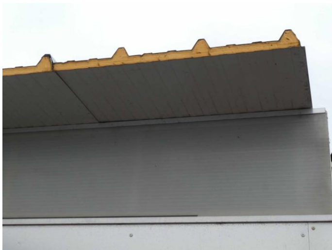
Figuur 23: Detail dak
