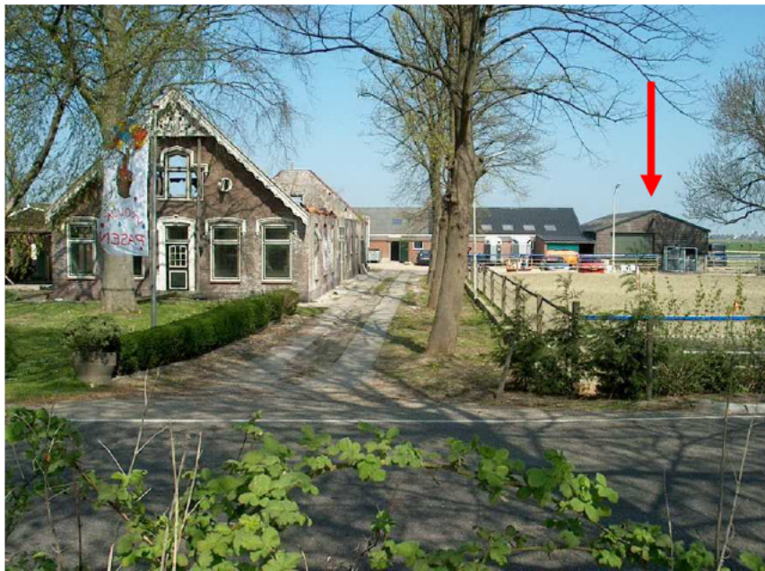
Foto 1: Te slopen loods
