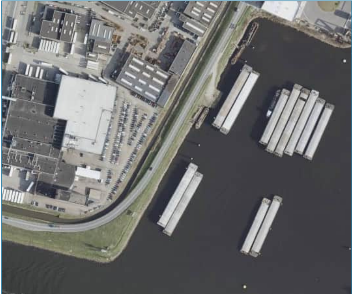
Figuur 3-1: De Gerrit Bolkade in 2021. (Cyclomedia)
