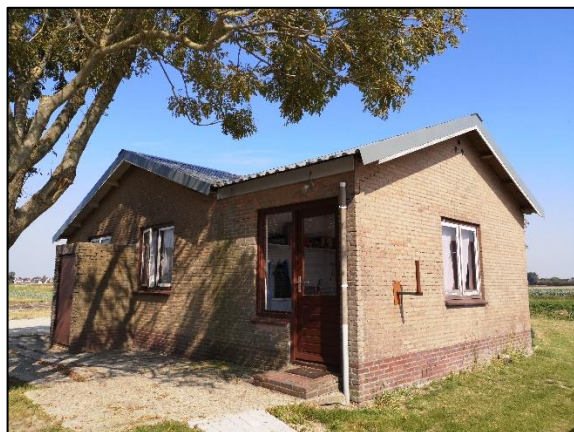
Afb 4: Te slopen woning
