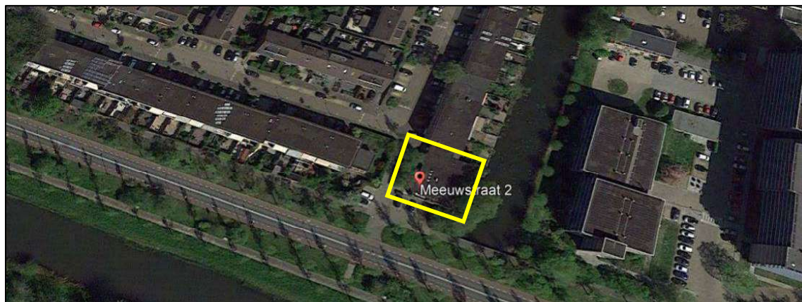
Afb 3: te slopen pand
