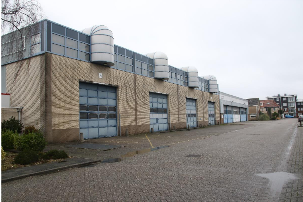
Gemetselde muren fabriekshal
