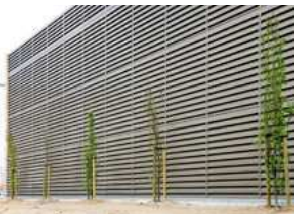
Parkeergarage in Osnabrück (DE)
