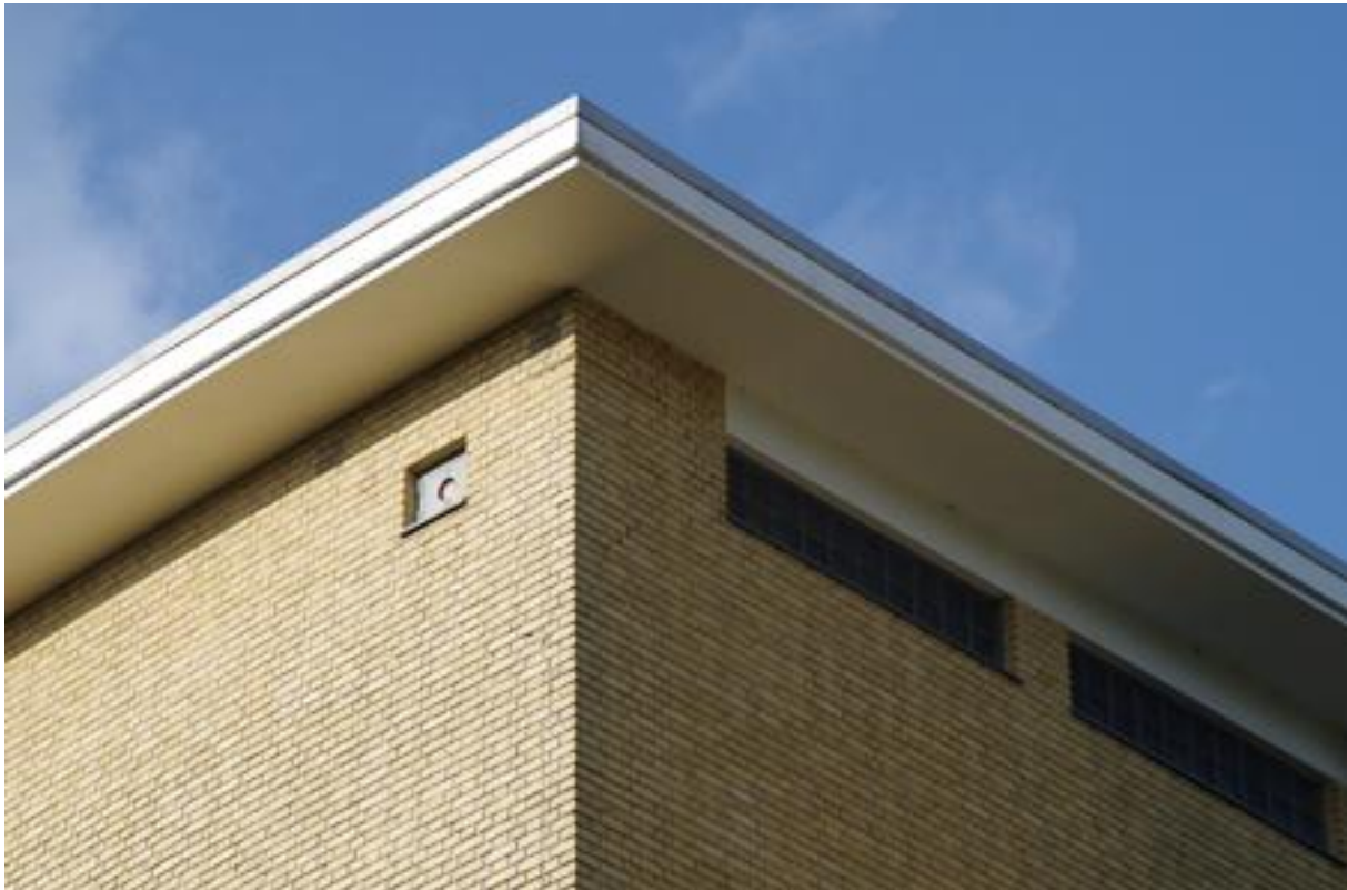
Detail gevel studio 2.
