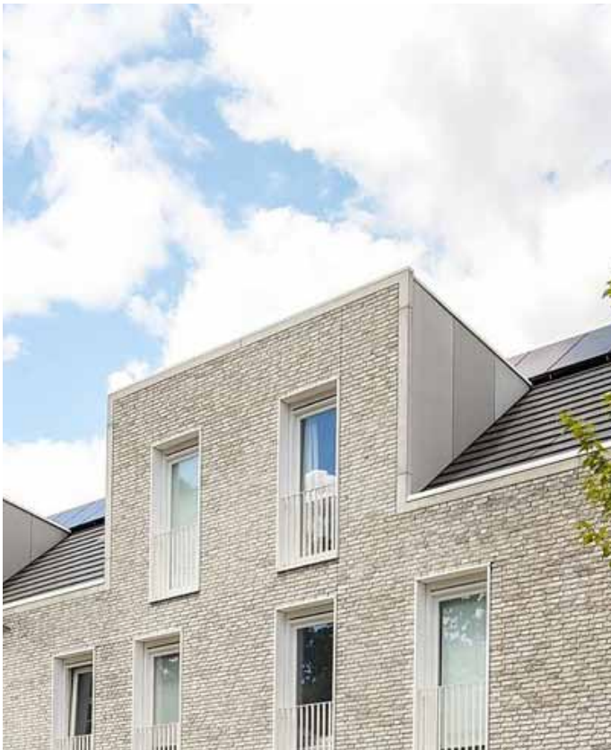
gemetselde 'dakkapel' in bovenste laag
