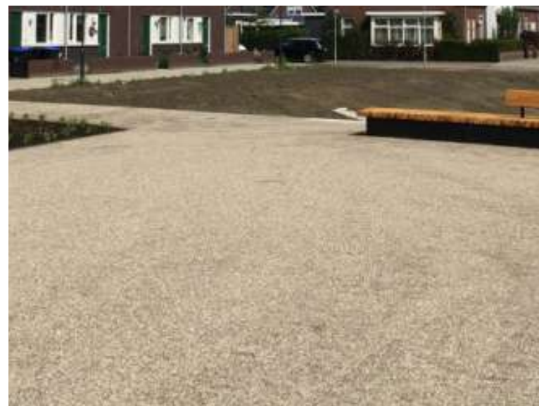
Stabilizer halfverharding IJsselmix (tbv boomspiegel)
