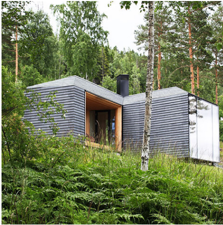
Cabin, Norderhov, Norway Atelier Oslo
