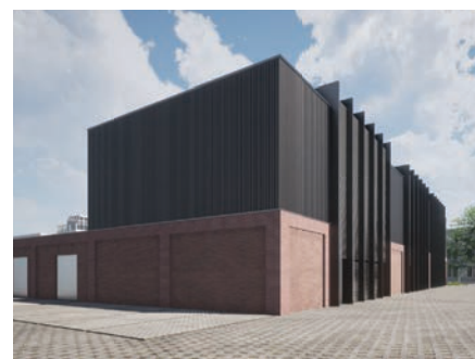
Transformatorstation IJburg, Amsterdam
