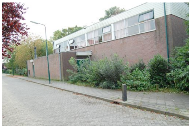
Te slopen gymzaal
