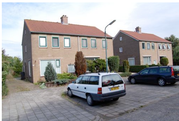
Te slopen woningen
