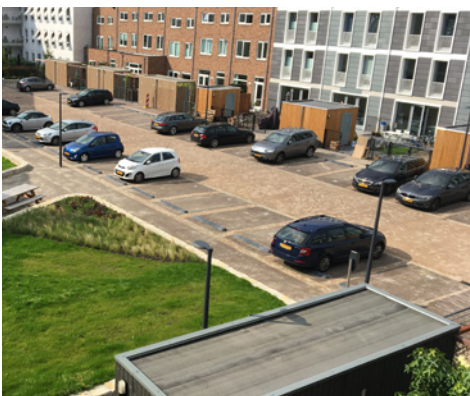
parkeren in binnenhof
