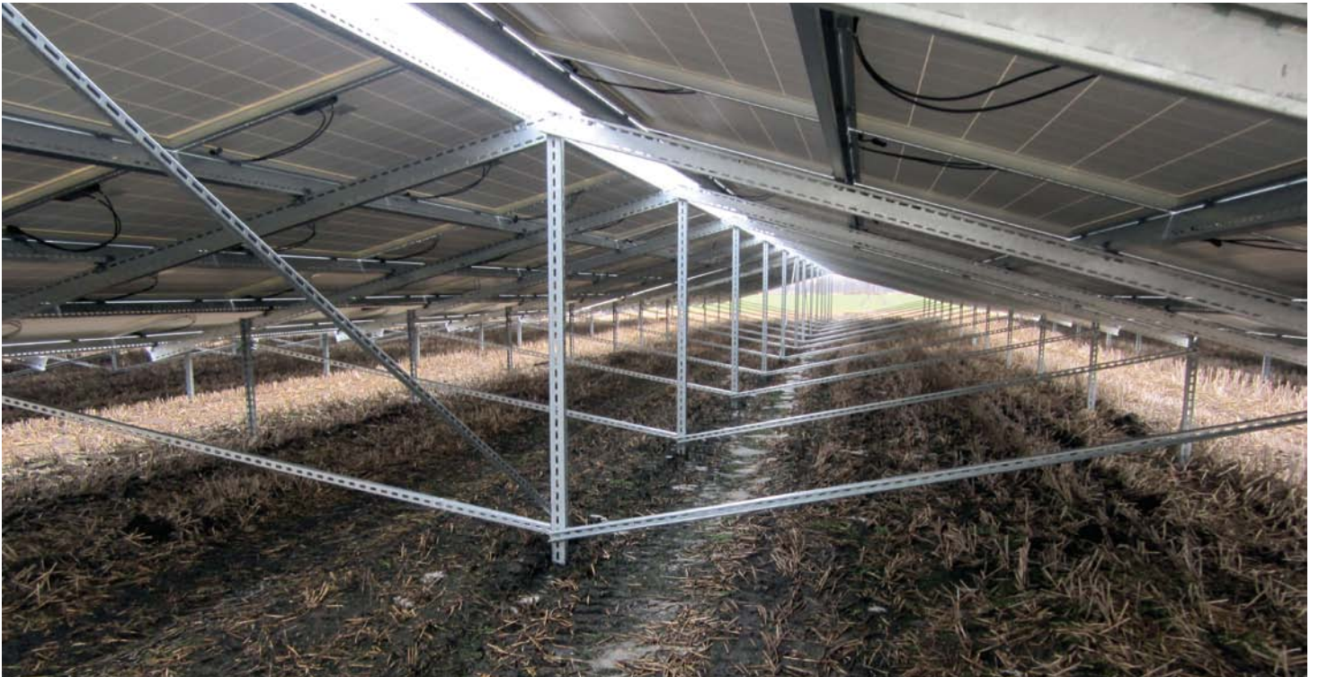
Modules, crystalline, 4-rows, landscape, east-west orientation
