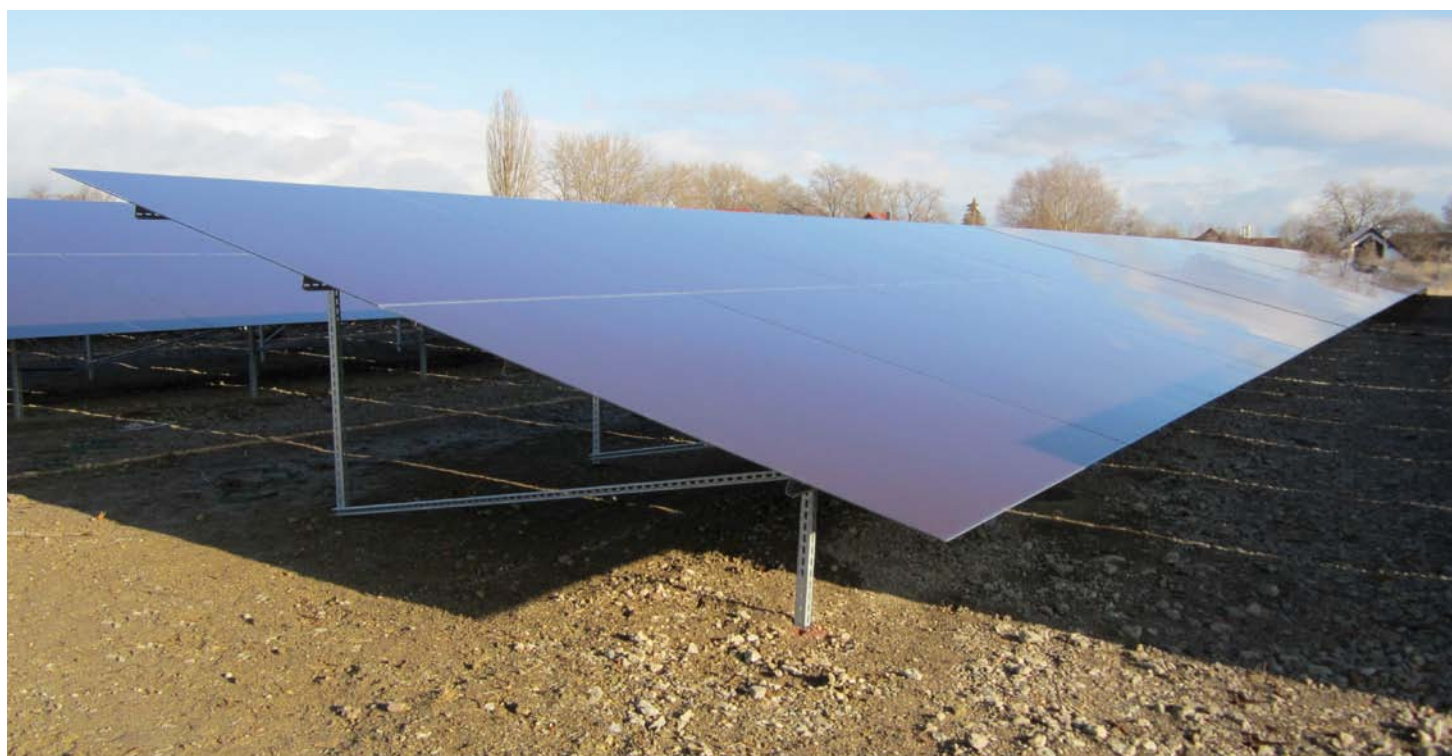
Modules, thin-film with back rails, 2.6 x 2.2 m, 2-rows, portrait
