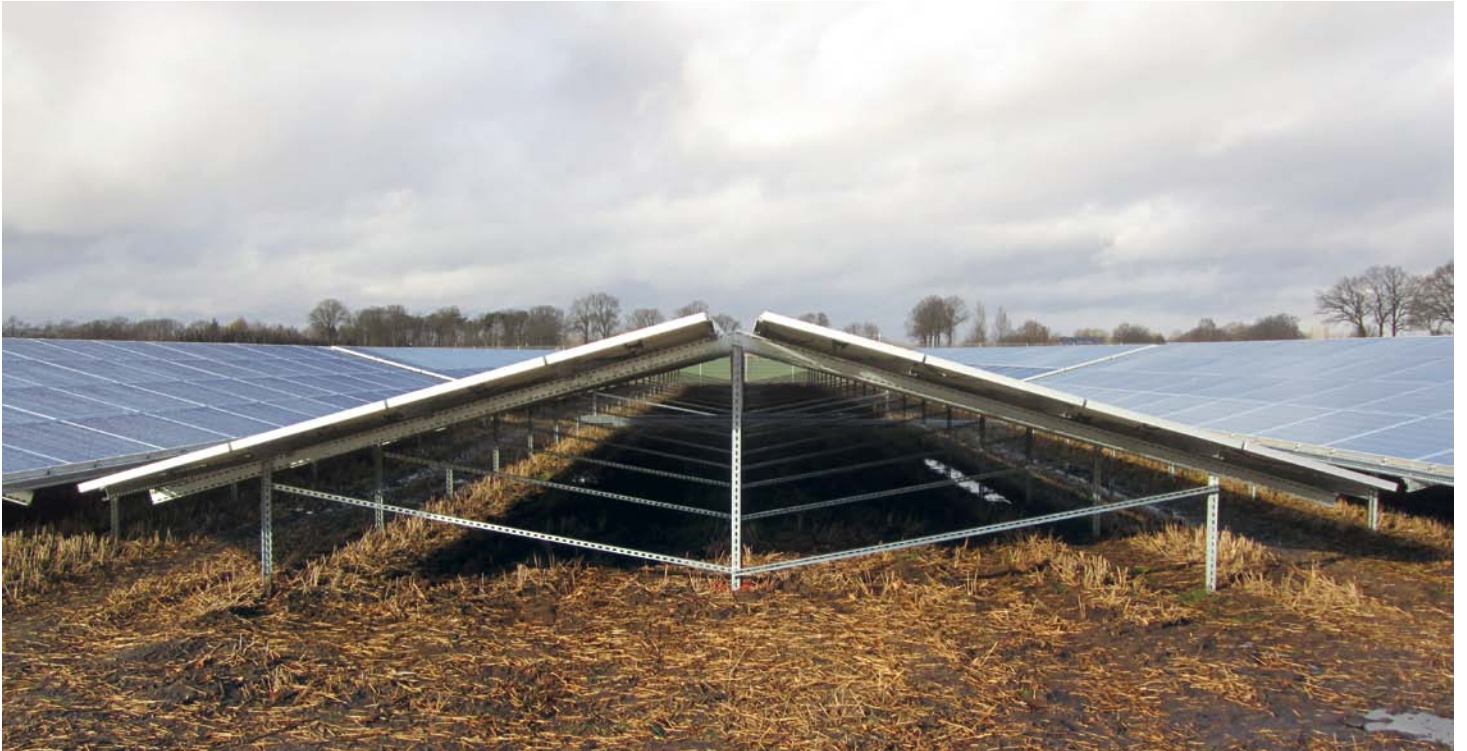
Modules, crystalline, 4-rows, landscape, east-west orientation
