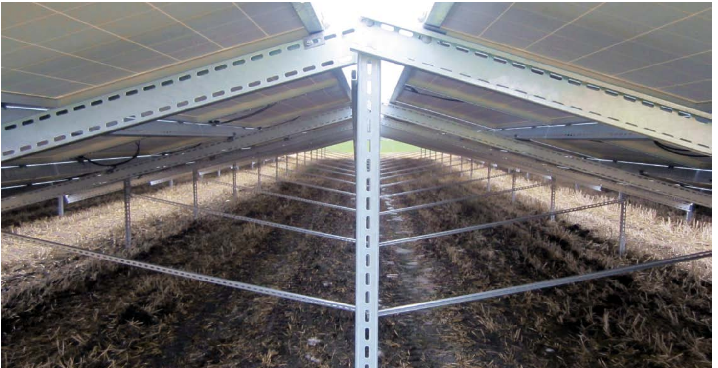
Modules, crystalline, 4-rows, landscape, east-west orientation
