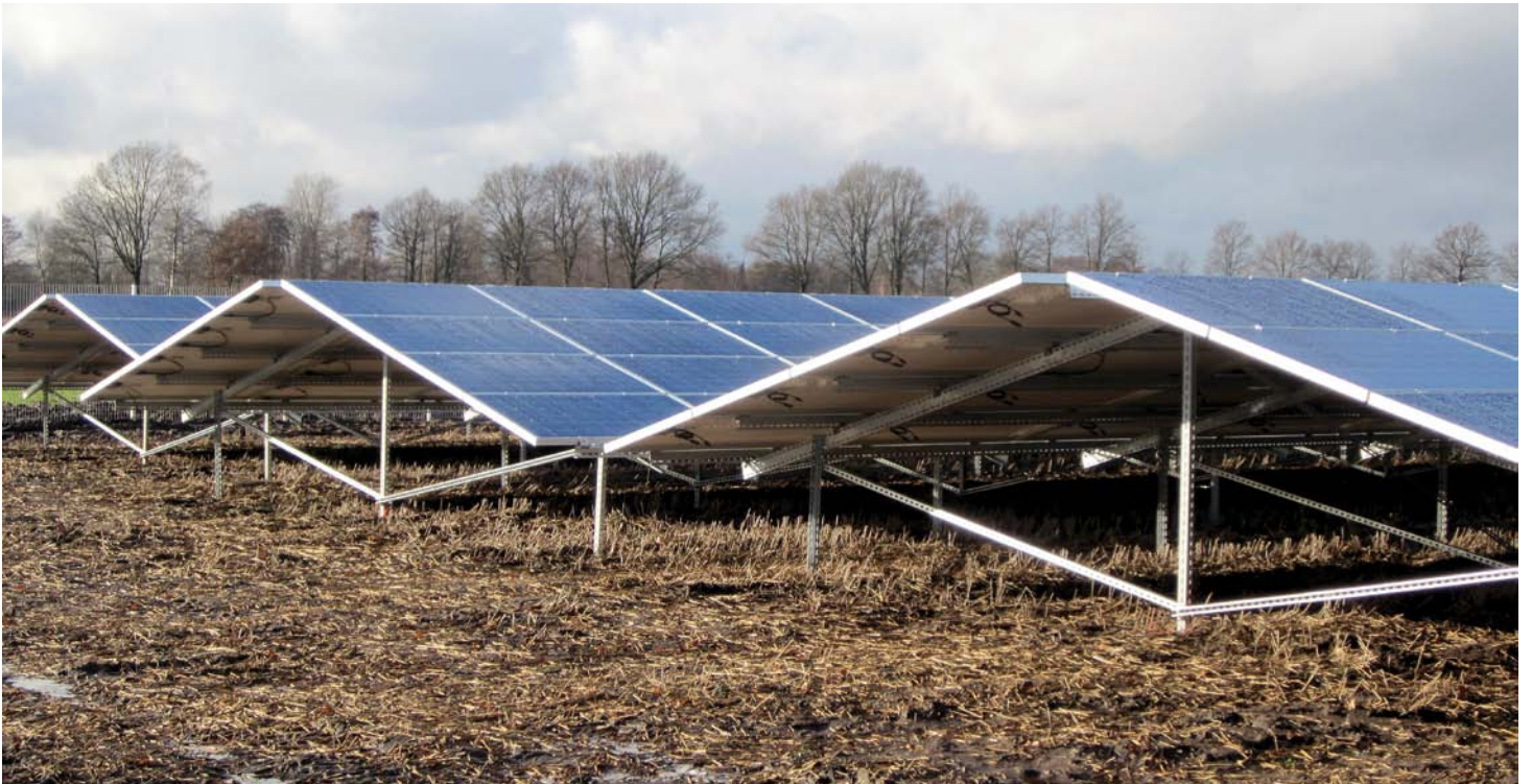
Modules, crystalline, 4-rows, landscape, east-west orientation
