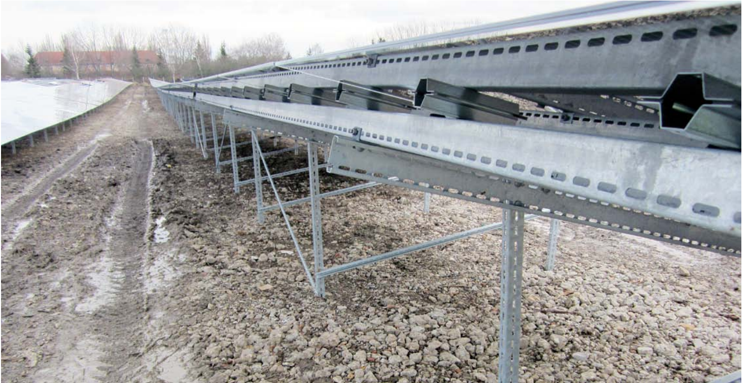
Modules, thin-film with back rails, 1.3 x 1.1 m, 3-rows, portrait
