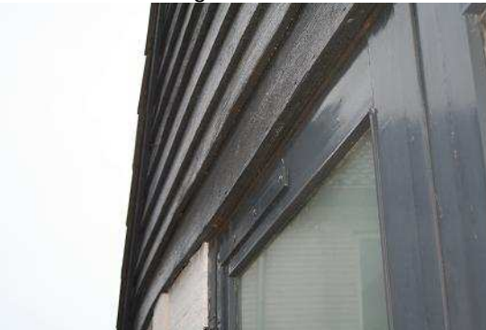
Detail betimmering loods.
