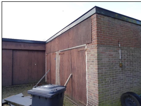
Fig. 2.3 Opstal 1 (bron: FF Solutions)
