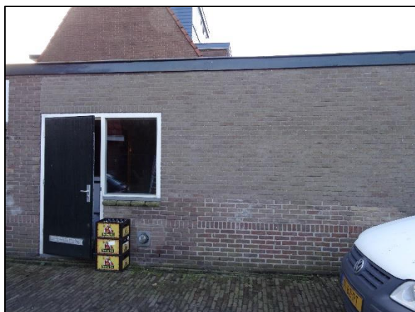
Fig. 2.2 Opstal 1 (bron: FF Solutions)
