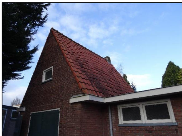
Fig. 2.6 Opstal 2 (bron: FF Solutions)
