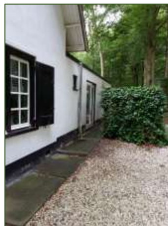
Fig. 2.7 Verhardingen rondom woning (bron: FF Solutions)
