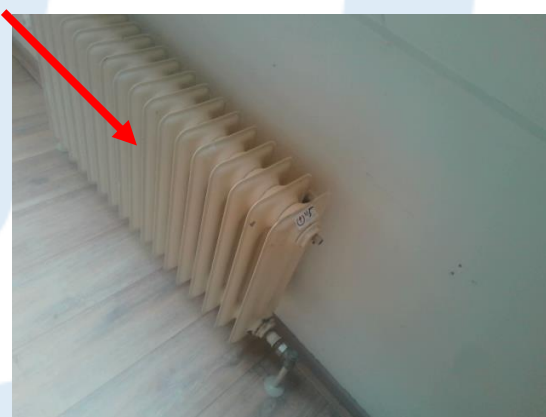
Foto 19 | Pakking lamellen radiator
