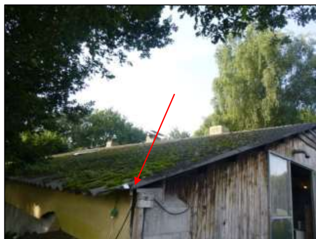
Foto 66: Schuur 3: Golfplaten dak incl. overlap & toebehoren (Bron 6) (Asbesthoudend)
