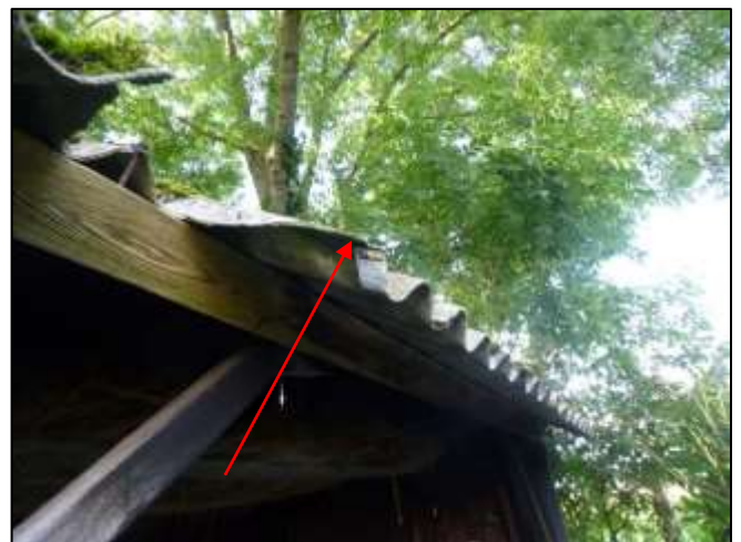
Foto 72: Schuur 4: Golfplaten dak incl. overlap & toebehoren (Bron 7) (Asbesthoudend)
