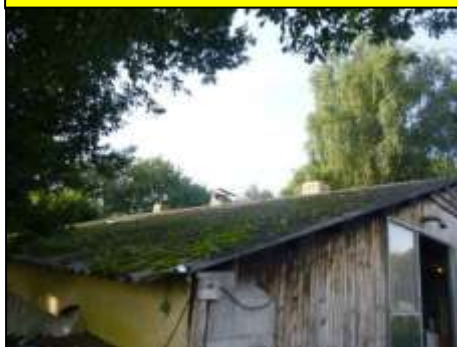
Schuur 3: Golfplaten dak incl. overlap & toebehoren (Bron 6) (Asbesthoudend)
