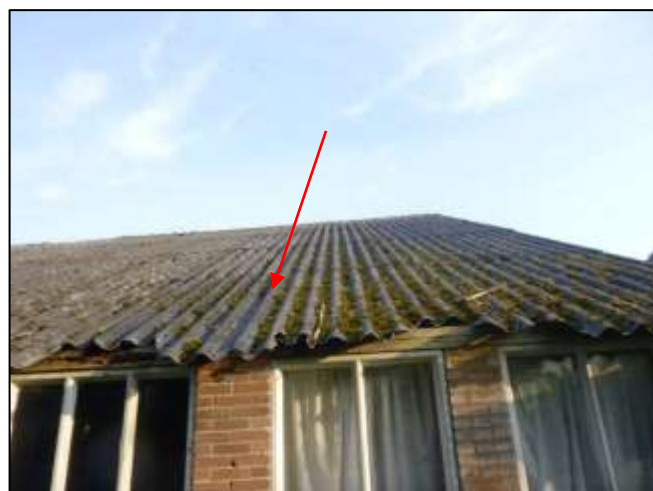
Foto 12: Schuur 1 & 2: Golfplaten dak incl. overlap & toebehoren (Bron 2) (Asbesthoudend)
