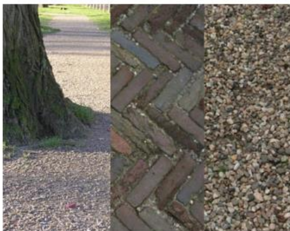
HALFVERHARDING - BESTRATING - GRIND
