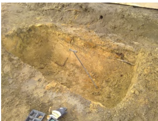
Foto 12 controle na tanksanering dmv olie-watertesten
