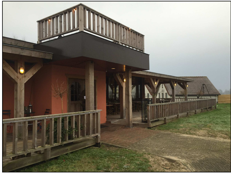
Foto 2 Restaurant Brandend zand
