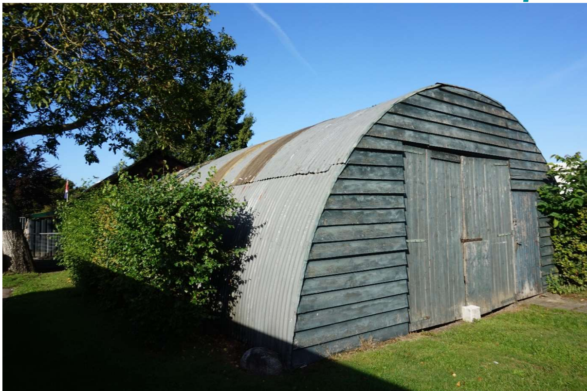
Figuur 2.4. Romney loods.
