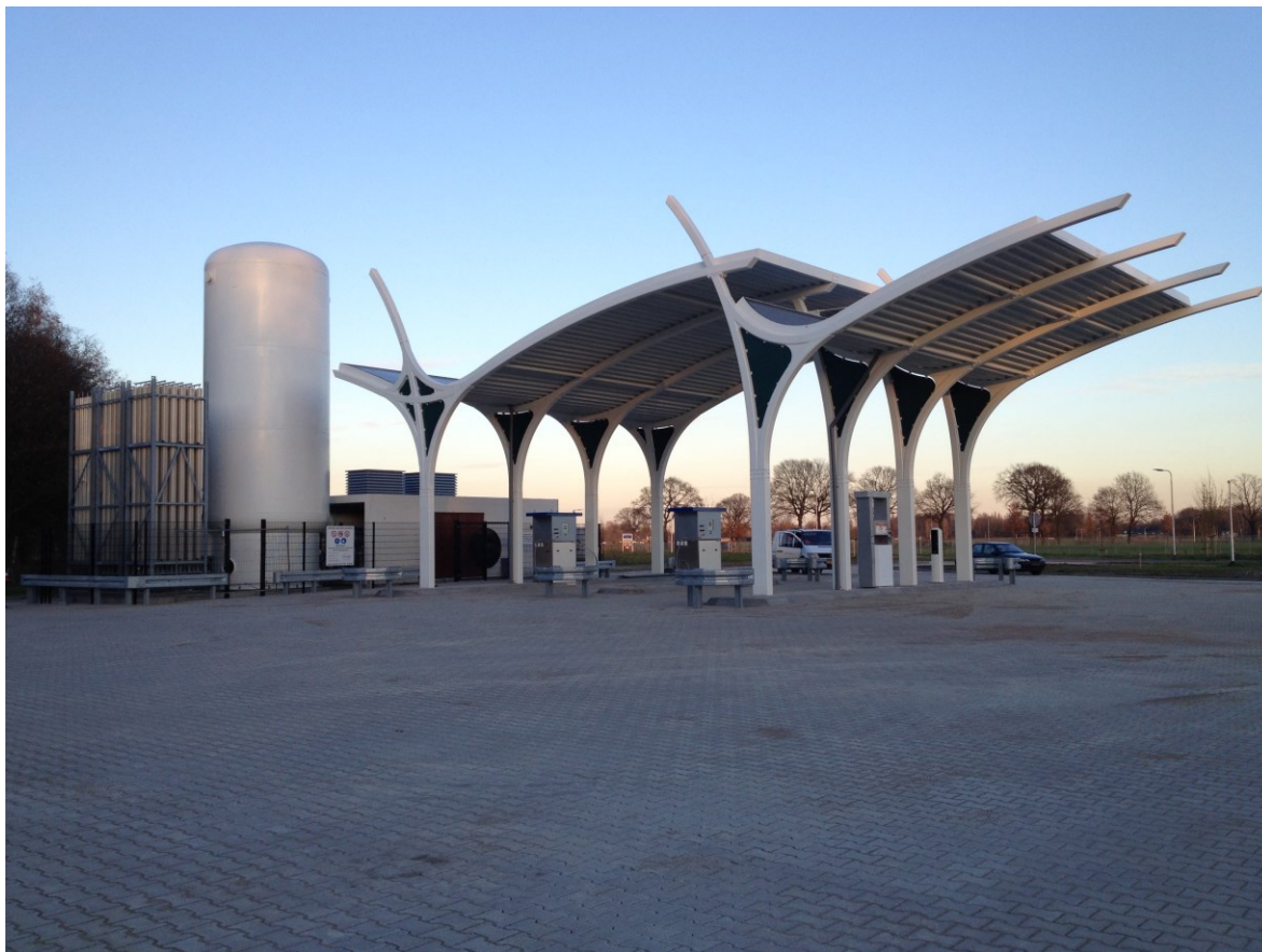
Foto 1: Bio-LNG tankstation “Schepersven” te Tilburg
