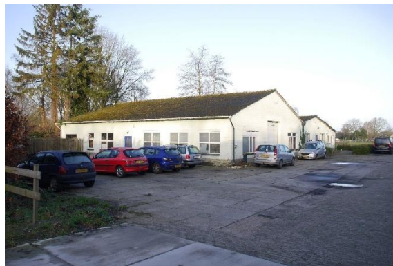
Foto 2: te slopen opstallen (foto Botani-Specialist)
