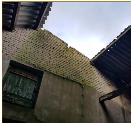
Afb. 2.11: Open dakbedekking in schuur 5.
