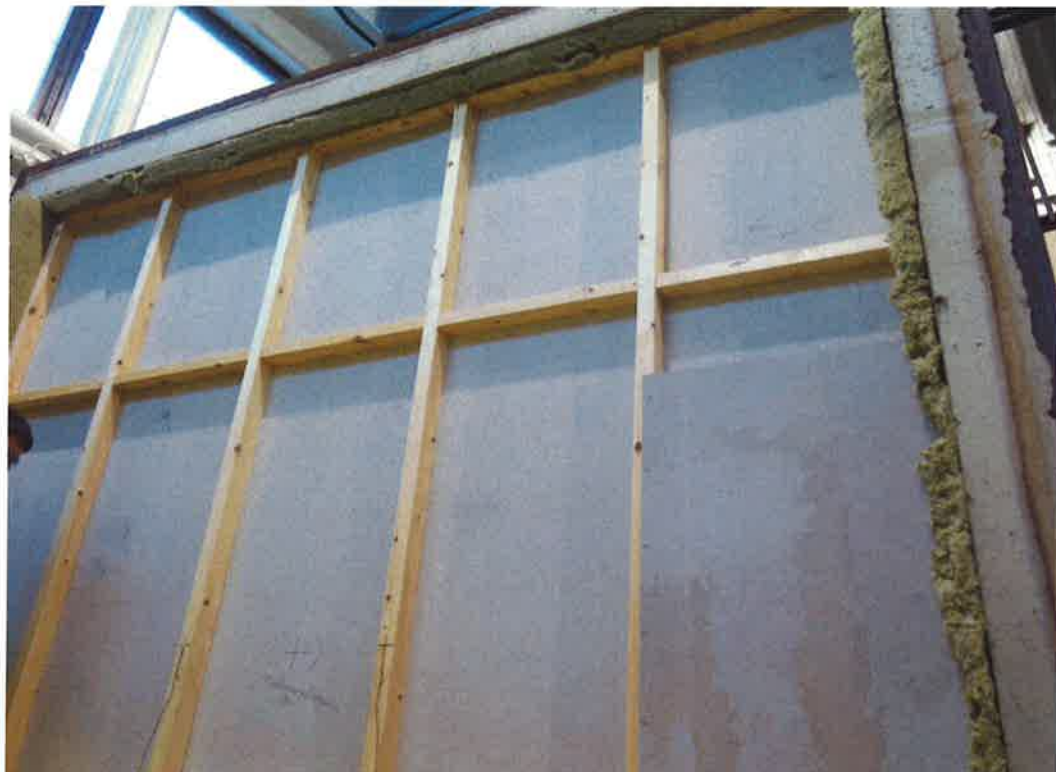
Figure 1. Fixing the wind shield boards on the exposed side of the studs
