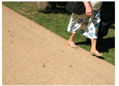
Halfverharding in gebroken split
