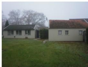
te slopen opstal 06-07
