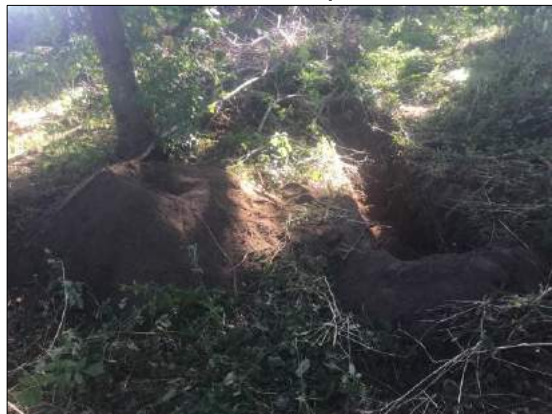
Foto 10: Sleuf SL07 (d.d. 21 september 2020)
