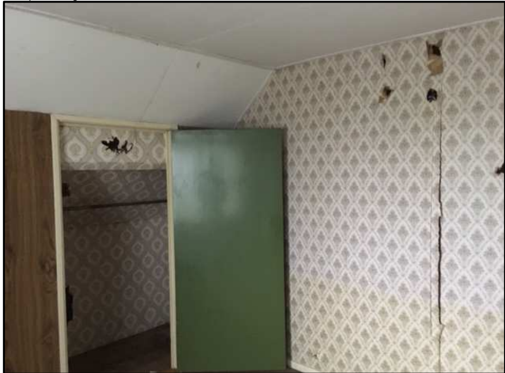
Te slopen woning kamers
