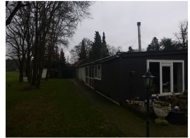
Verharding rondom appartement in meubelzaak
