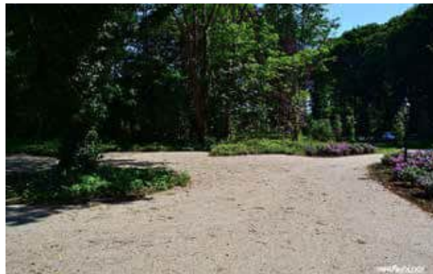
Halfverharding ( Durecomix/gelders padvast)
