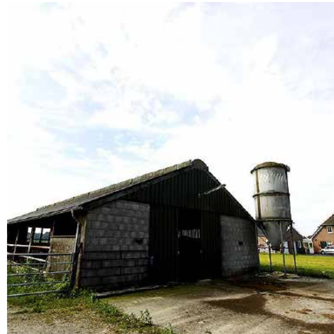
te slopen stal Schaddenveldsweg
