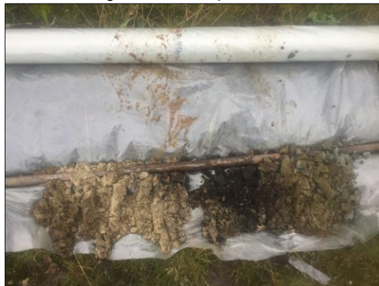
Foto 10: Boring 11 (d.d. 01 september 2020)
