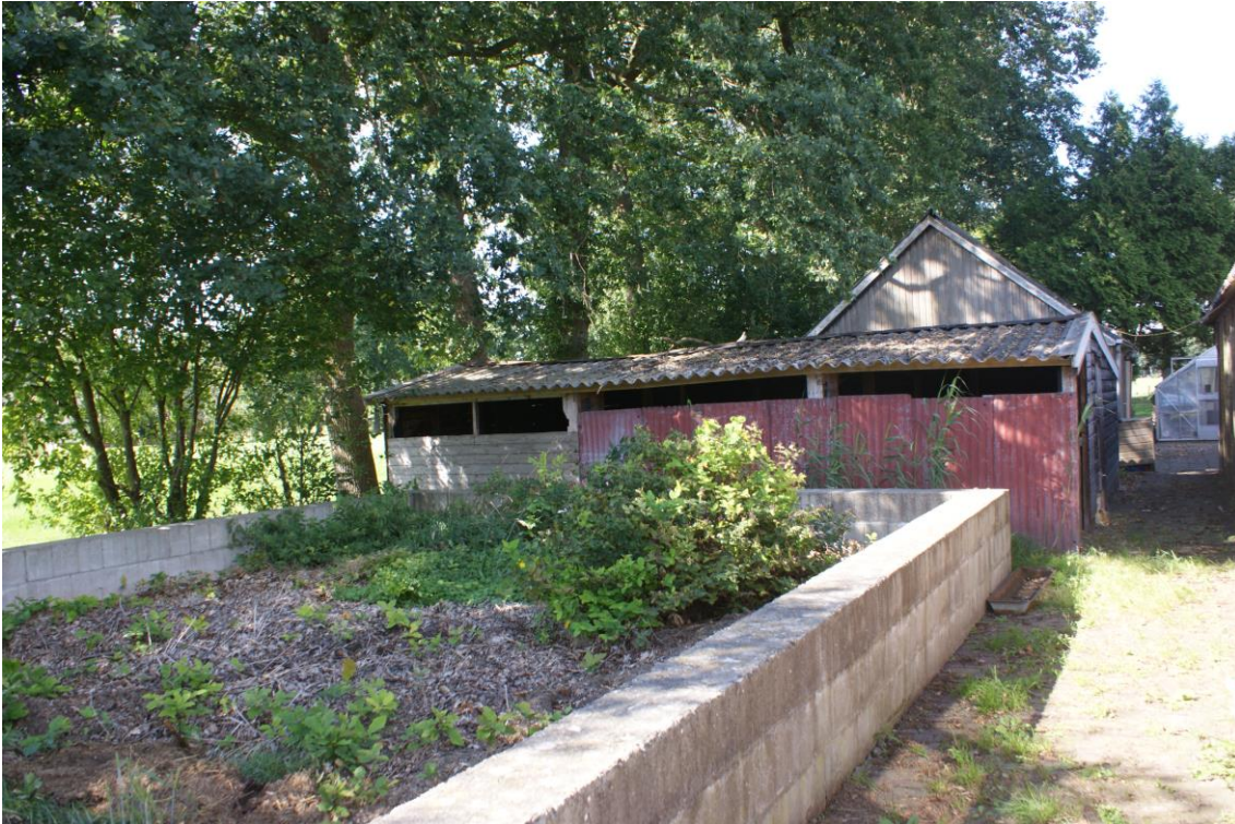
Fig. 2.4 Te slopen garage
