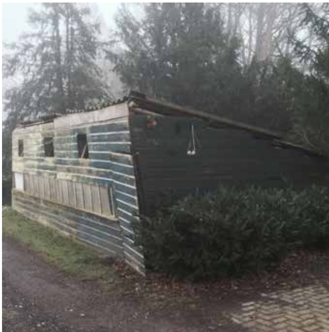
te slopen kippenstal
