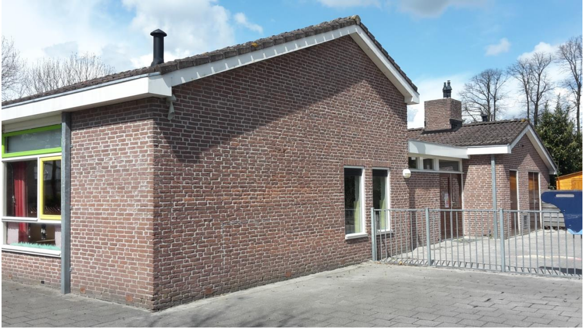
Figuur 1.2: De te slopen school, Villa Kakelbont.
