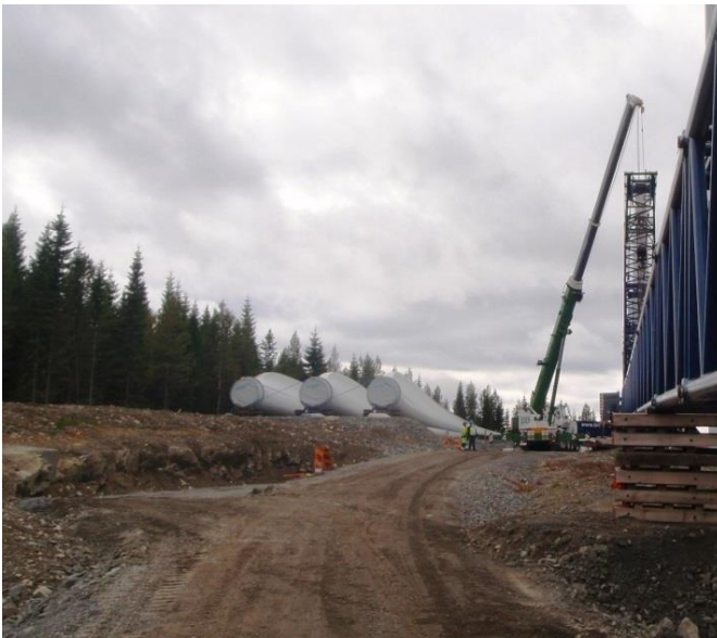
Figure 13: Example of Hardstand for Assist Crane q2 on hilly terrain. Despite of the gradient of adjoining road, q2 must always be levelled to within 1.5%.
