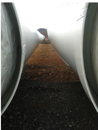
Figure 19: Example of a well prepared area between blade fingers.
