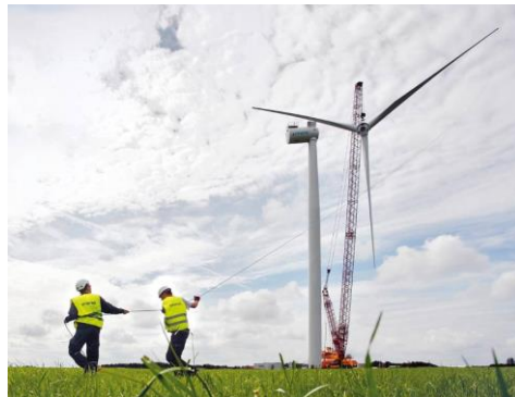
Figure 28: Tag line for rotor installation.
