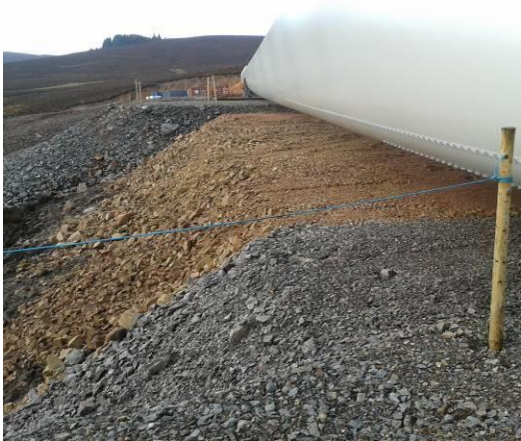
Figure 17: Example of trestle area q4
