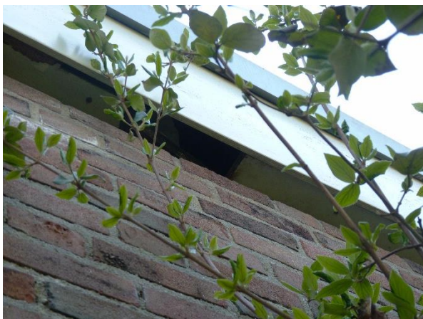
Foto 15 Openingen in holle dakrand
