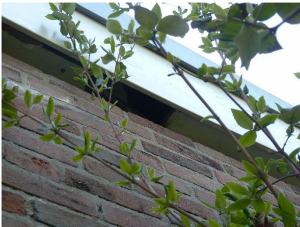
Foto 15 Openingen in holle dakrand
