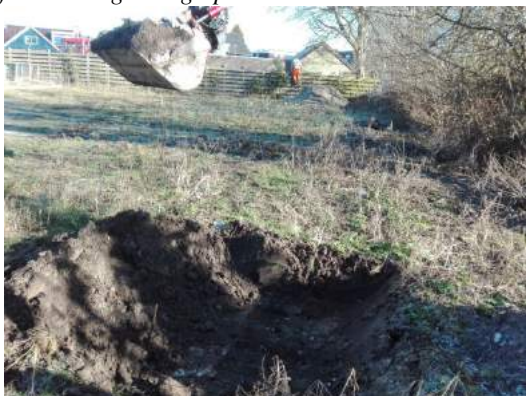
foto 5: ontgraving Spot C
