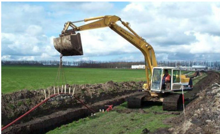
Figure 10: Typical crane with a quadrant
