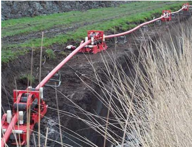
Figure 8: Typical cable tensioners
