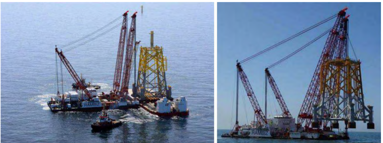
Figure 58 Installation of jacket
