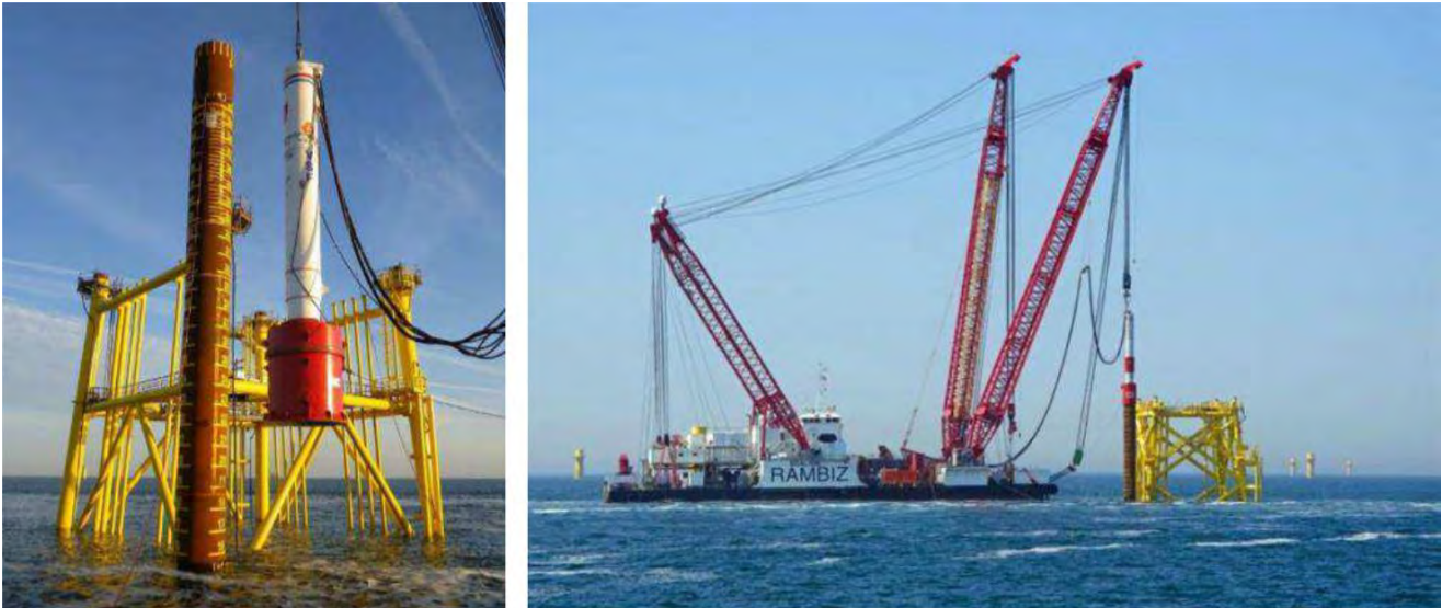
Figure 59 Piling of jacket
