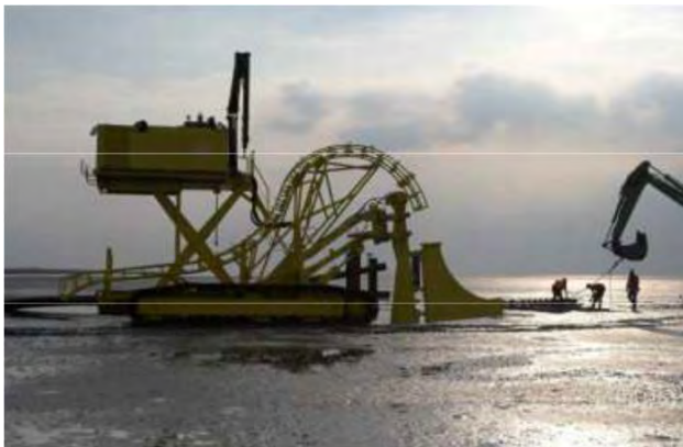
Figure 51 Vibration plough on tracks
