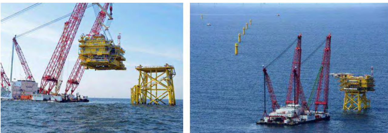
Figure 60 Installation of topside
