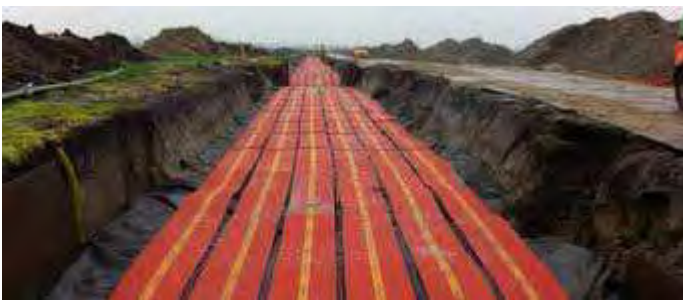
Figure 18 Open cable trench, after the pull-in of the cables
