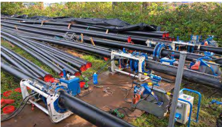
Figure 27 Welding of HDPE ducts
